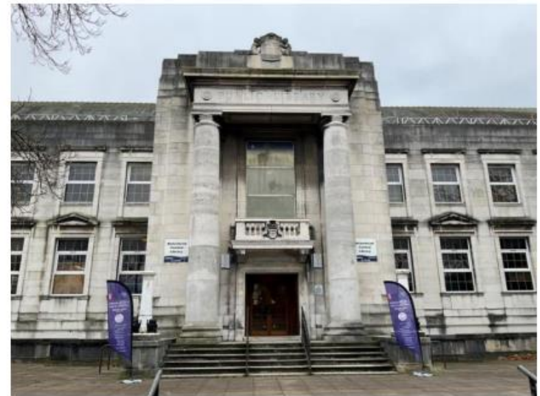
Main entrance view of Birkenhead Central Library showing solid wall construction
