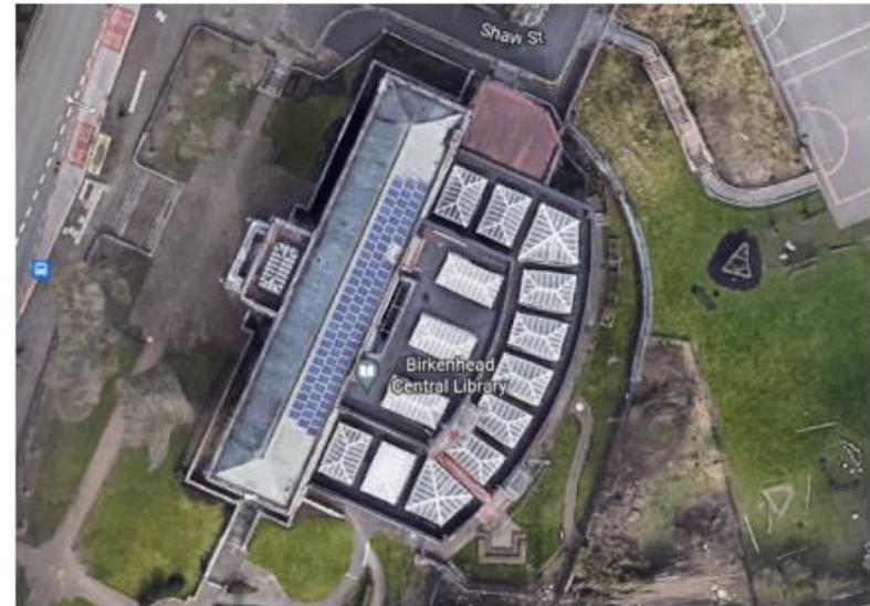
Aerial view of Birkenhead Central Library showing the existing solar panels
